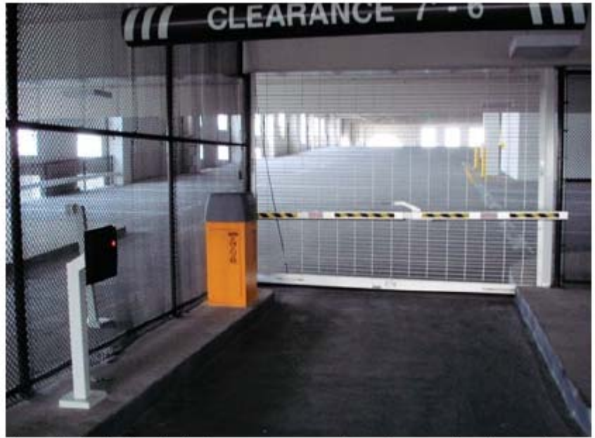
The top level of a three-level parking garage at Veranda Park is accessible only to residents who pass through gates using HID Global proximity technology. The garage is also secured with emergency call stations and multiple video surveillance cameras on each level.
